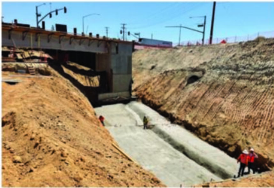
Crews working on the future retaining wall system where the lowered Jurupa Rd. will be constructed.
