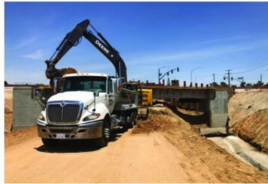
Crews working on the future retaining wall system where the lowered Jurupa Rd. will be constructed.
