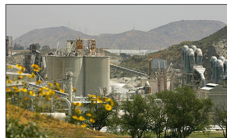
Figure 6-8: Former Riverside Cement Company plant, Jurupa Valley
