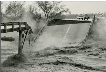
Figure 4-11: Van Buren Bridge collapse during 1969 Santa Ana River flooding
