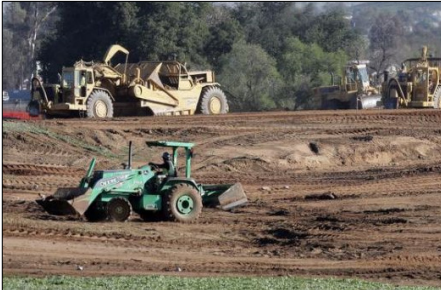
Figure 7-11: Construction graders, Inland Empire
