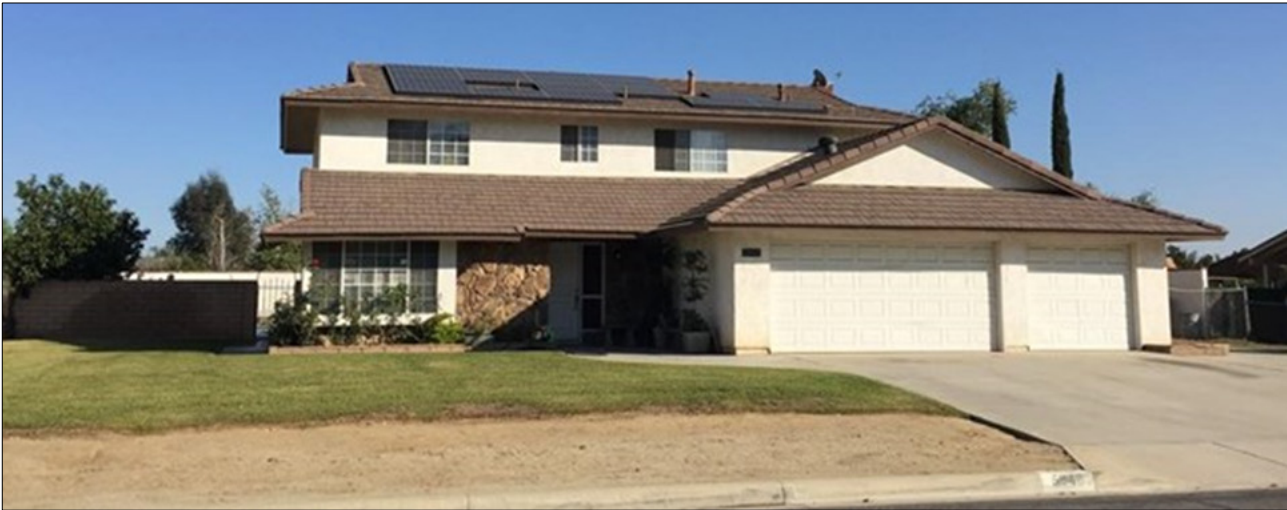
Figure 4-14: Residential roof-mounted photovoltaic solar collectors
