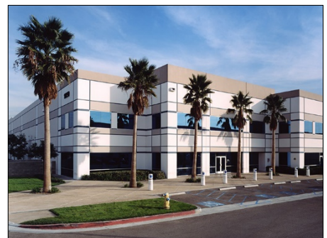
Figure 11-4: Logistics building, Jurupa Valley
