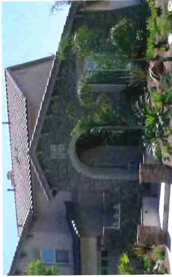
Material Break - stucco / stone
