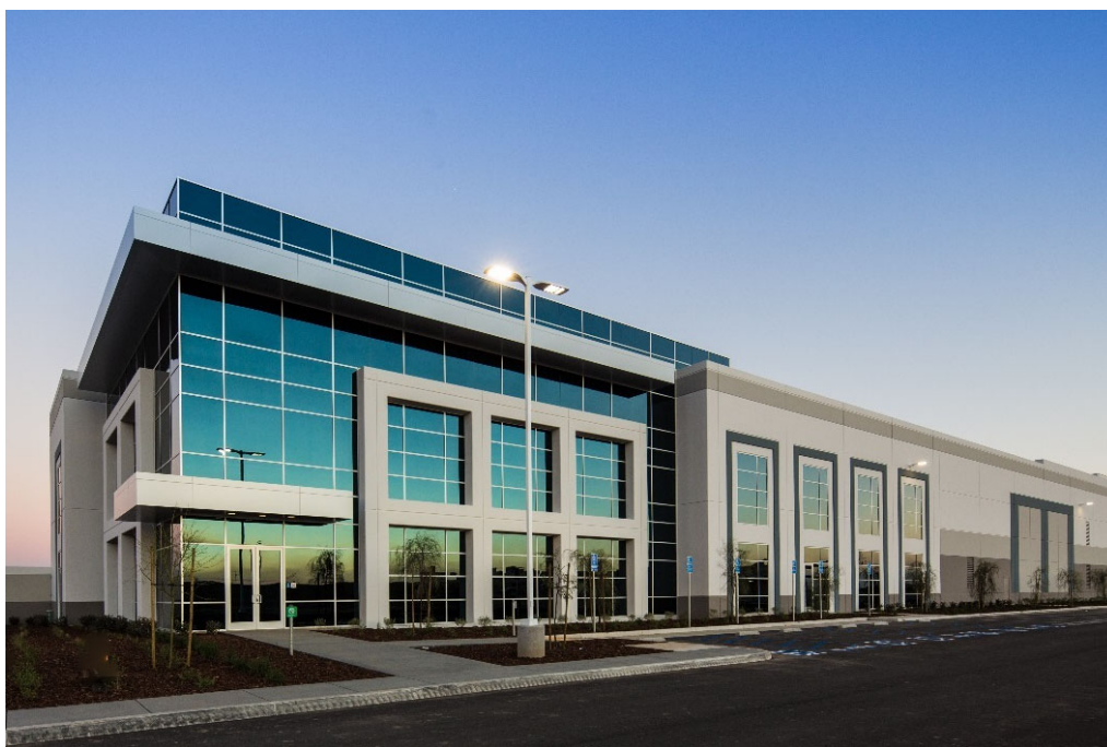
Contemporary light fixtures provide an attractive, safe working environment.
