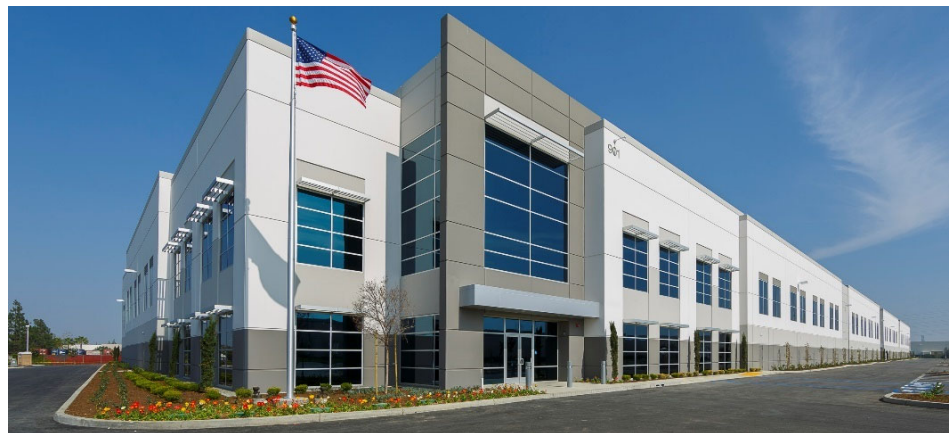
Window design creates a horizontal emphasis and frames the primary building entry.
