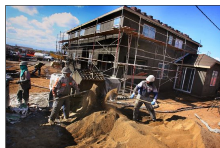
Figure 5-4: Housing construction in Jurupa Valley
