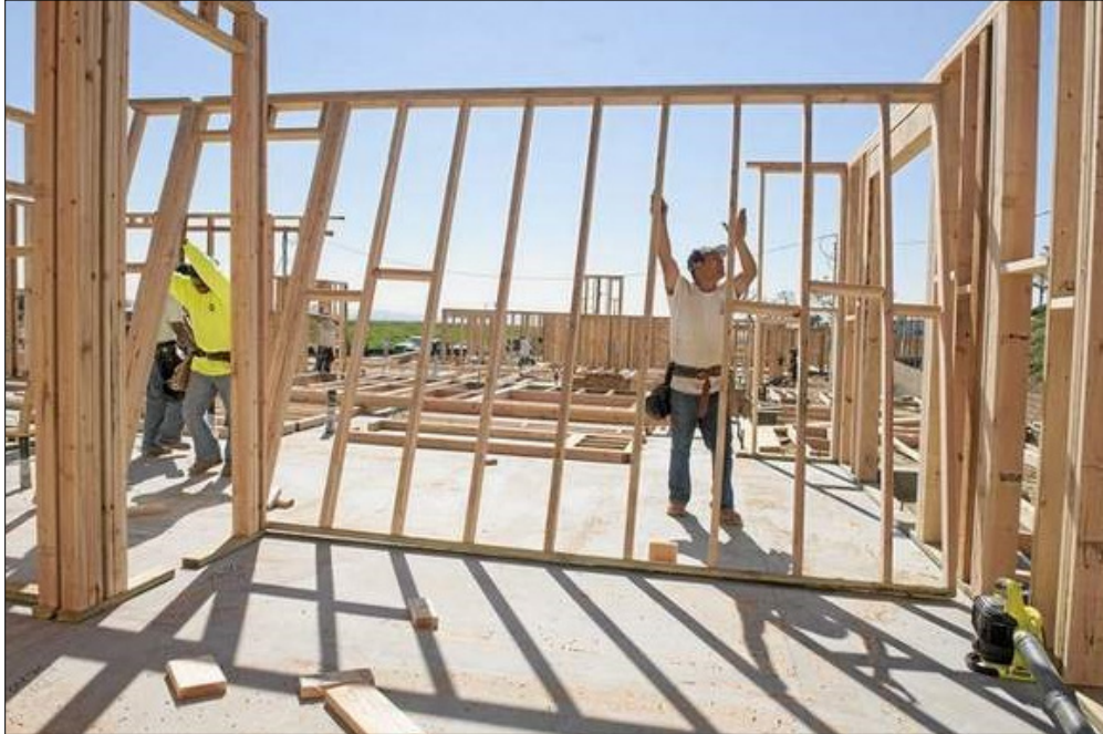
Figure 5-1: New housing construction in Jurupa Valley
