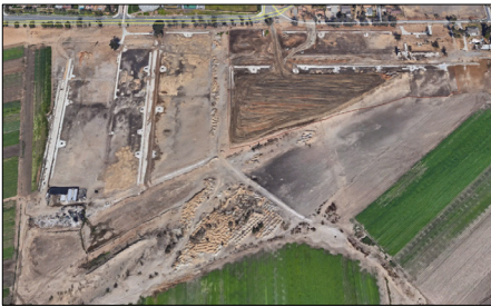
Figure 5-2: Subdivision under construction, Jurupa Valley
