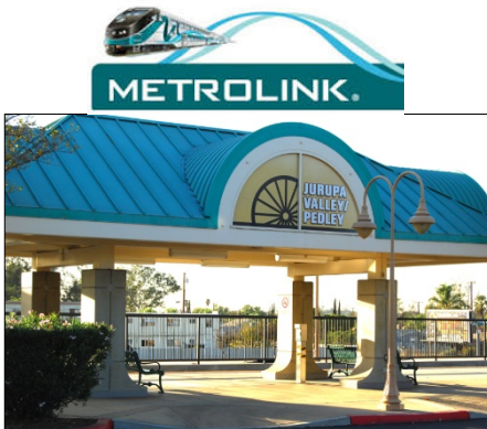
Figure 3-20: Metrolink station in Jurupa Valley
