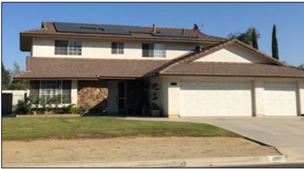
Figure 6-9: House with photovoltaic solar panels
