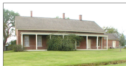
Figure 4-17: Historic Jensen-Alvarado Ranch House, 1870
