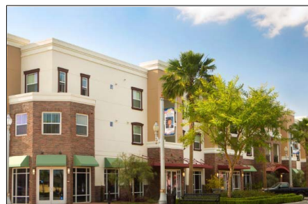
Figure 2-26: Mixed use senior housing over retail commercial, Riverside County (KTGY Architects)
