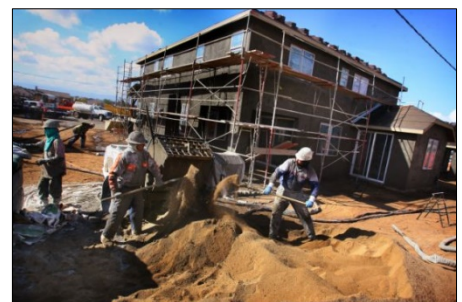
Figure 11-3: New housing under construction near Vernola Marketplace
