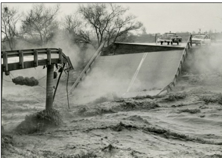
Figure 8-7: Van Buren Bridge collapse during the 1969 Santa Ana River flood (Riverside County Flood Control and Water Conservation District)
