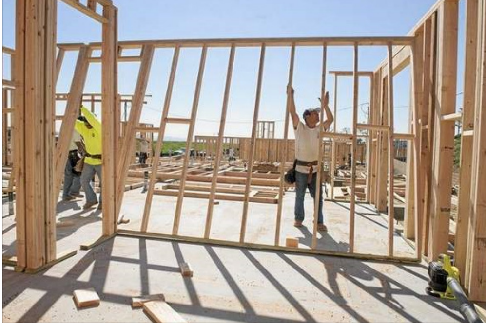
Figure 5-1: New housing construction in Jurupa Valley
