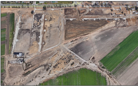
Figure 5-2: Subdivision under construction, Jurupa Valley
