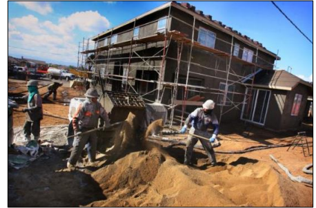
Figure 5-8: Housing construction in Jurupa Valley
