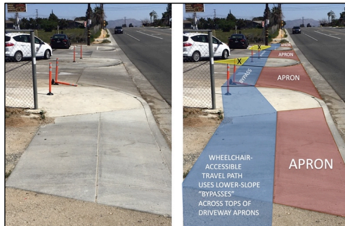
Figure 4-23: Limonite north sidewalk across El Torito driveways
