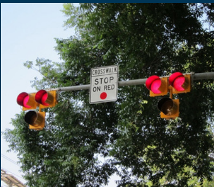
Example of PHBs mounted on a mast arm. Source: FHWA
