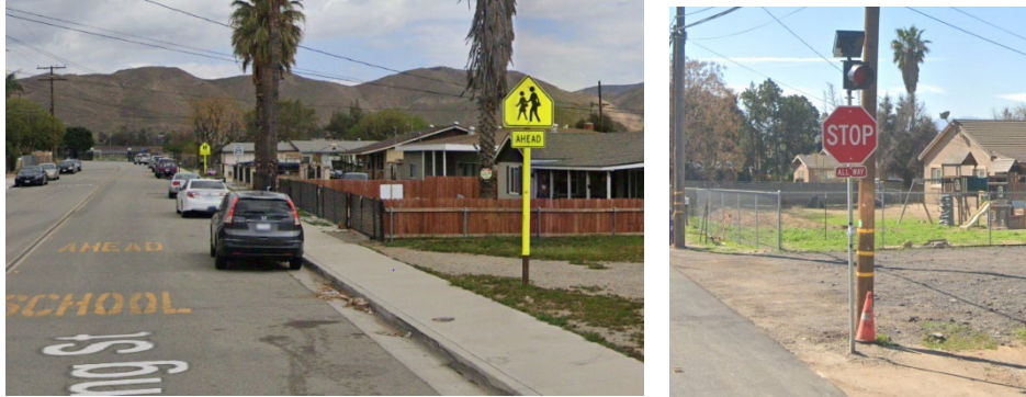
Reflective Signpost Covers and Pole-Top Flashers for Enhanced Sign Visibility
