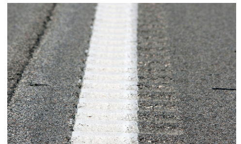
Example of an edge line rumble stripe. Source: Missouri DOT
